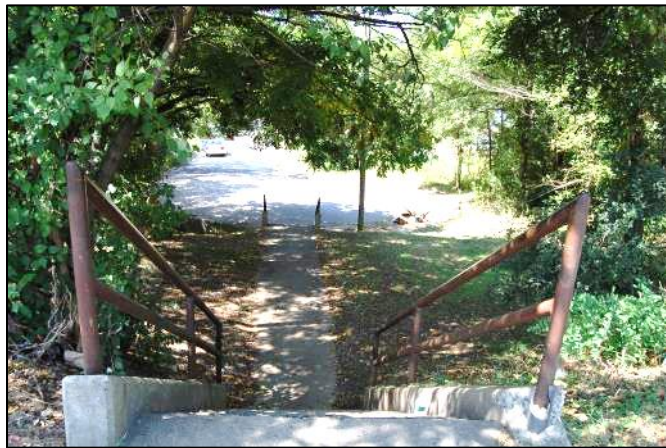
Figure 13. Steps put in, during construction of East-West Expressway, from South Alston Avenue down to new cul-de-sac at east end of Jacob Street
